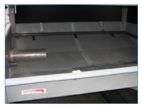
A sump sweeper piping system **increases water circulation and agitation** in the basin and is designed to be used in combination with a <u>filtration</u> system. It does all this:
