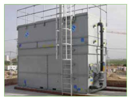
A ladder, safety cage and handrails are all installed for **easy access to the unit top and easier and safer** inspection and maintenance, in line with **EU safety directives**. For units equipped with these options, we also recommended installing <u>steel drift eliminators</u>.
