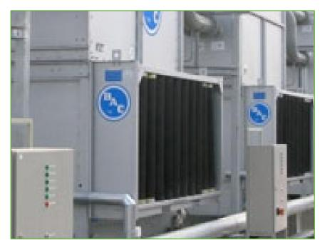
FXVS closed circuit cooling towers use **quiet and low kW axial fans**, but to reduce noise even further, you can extend your FXVS cooling tower with sound attenuation:
