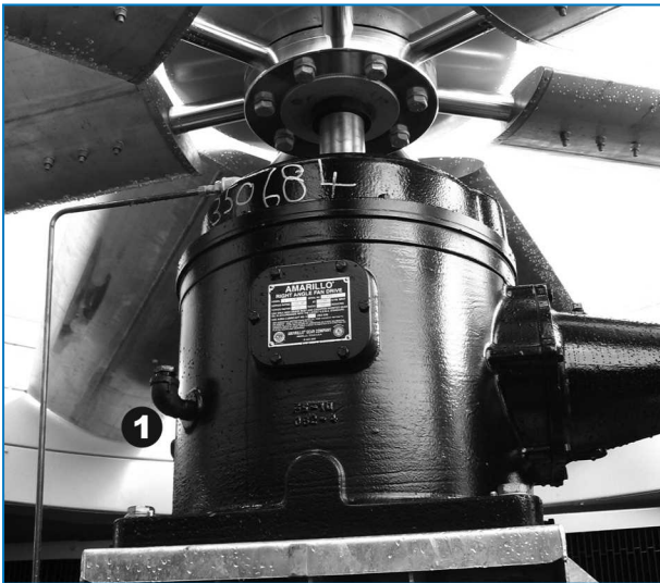
Single reduction gear drive
