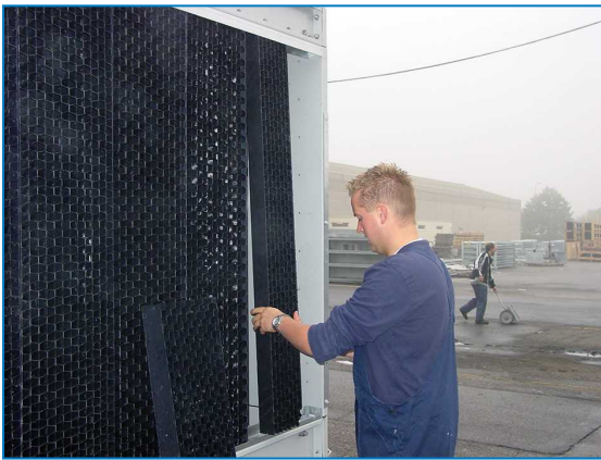
Remove combined inlet shields
