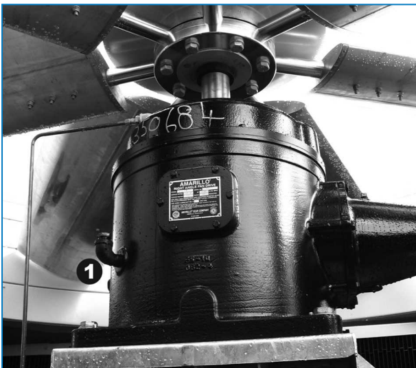
Single reduction gear drive
